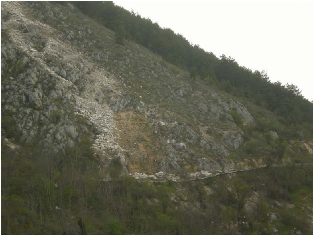
Figura 42 Pareti di distacco e grossi massi calcarei crollati (WPT RN10 42.3171/13.4705). Figure 42 Surface of detachment and mass fall (WPT RN10 42.3171/13.4705).
