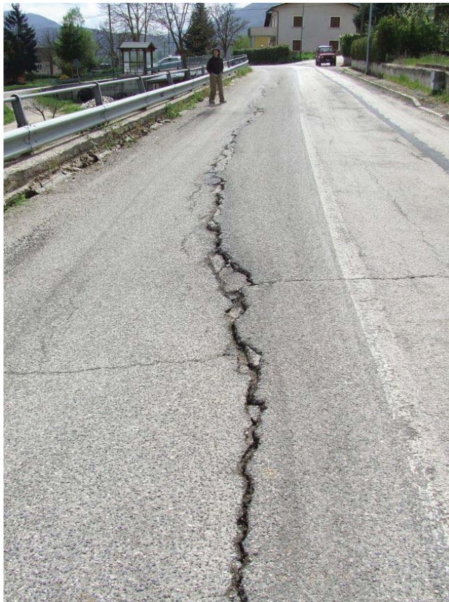
Figura 47 Frattura lungo la strada Casentino-Tussillo (WPT RN15, 13.5312/42.2692). Figure 47 Break in the paved road Casentino-Tussillo (WPT RN15, 13.5312/42.2692).
