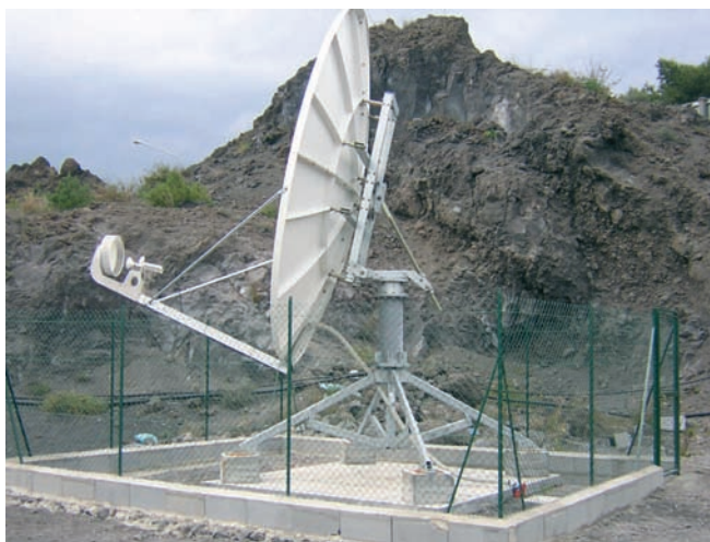
Figura 36 Antenna parabolica da 3.8 m, installata presso la sede CUAD di Catania. Figure 36 Satellite dish, 3.8 m, installed at the CUAD base in Catania.
