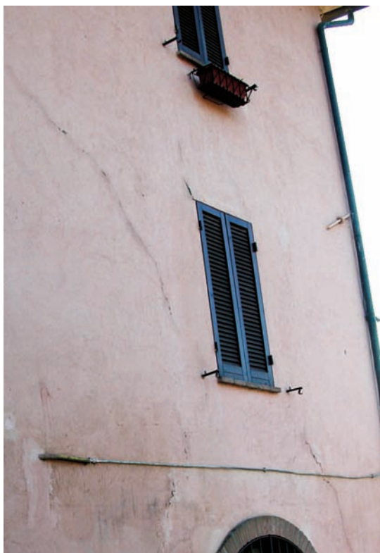
Foto 12 Pieve Caina (Marsciano, PG), lesioni leggere ( dt ). Photo 12 Pieve Caina (Marsciano, PG), slight cracks ( dt ).
