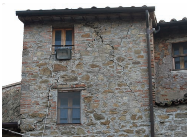
Foto 4 Spina (Marsciano, PG), crepe larghe e profonde ( d3 ). Photo 4 Spina (Marsciano, PG), large cracks in the wall ( d3 ).
