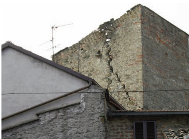
Foto 3 Spina (Marsciano, PG), importante cedimento ( d4 ) in edificio fatiscente. Photo 3 Spina (Marsciano, PG), serious failure ( d4 ) in a bad maintained building.
