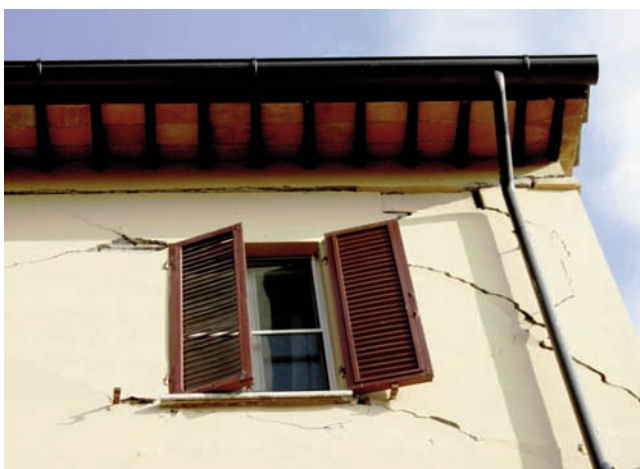
Foto 5 Spina (Marsciano, PG), crepe larghe e profonde (d3). Photo 5 Spina (Marsciano, PG), large and extensive cracks (d3).
